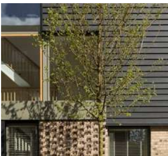
Contrasting brick / vertical boarding.
